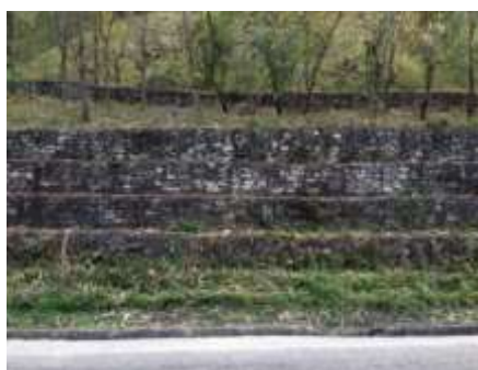
(e) Gabion Wall
