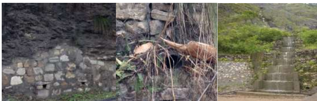
(a) Stone Masonry Wall with Weep Holes for Drainage
