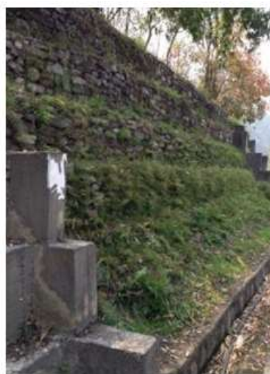
Fig. 5. Bio-engineering (Vegetation Plantation) in Krishna Bhir Slope.
