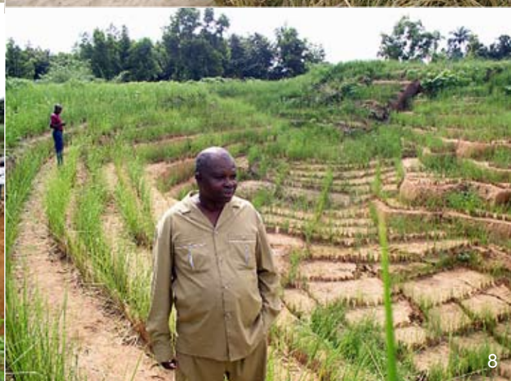
Figures 3- 4. Use of new plantings of Vetiver Grass to stabilize slopes bordering a new railway in northern Madagascar. 3, Low-lying portion; 4, Elevated portion. (Photographer: Yoann Coppin ).
